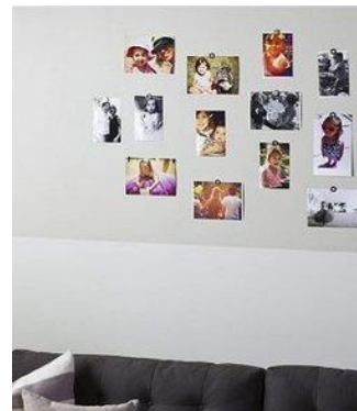
Linoleum pin-board integrated in wall
